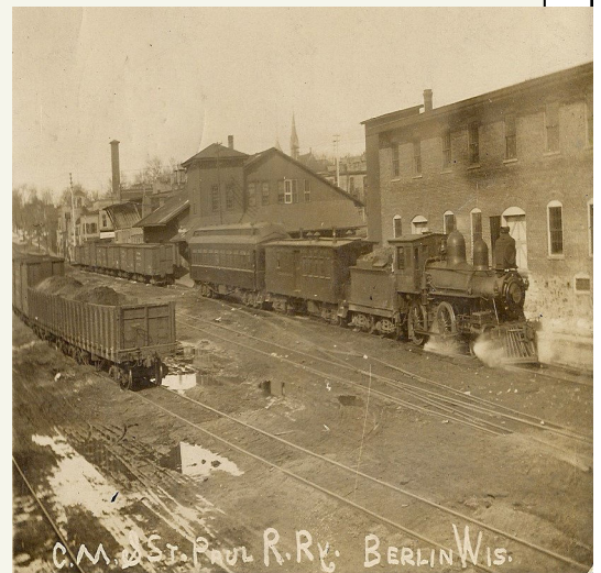
South Capron St. Rail Yard
